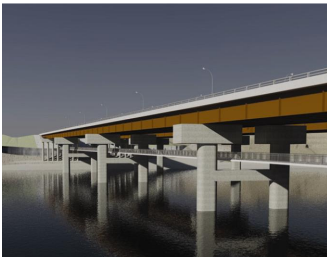
The 304-metre North Saskatchewan crossing will include a pedestrian/cyclist bridge located under the south bridge.
